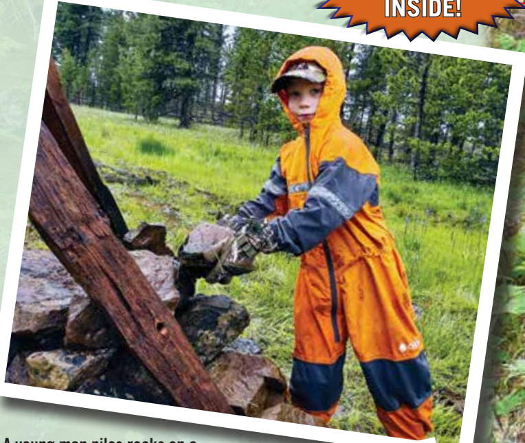
A young man piles rocks on a rock jack that helps hold up the corners of a fence.
